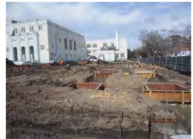
Eleanor L. McMain Gymnasium Piling and Pile Caps Completed
