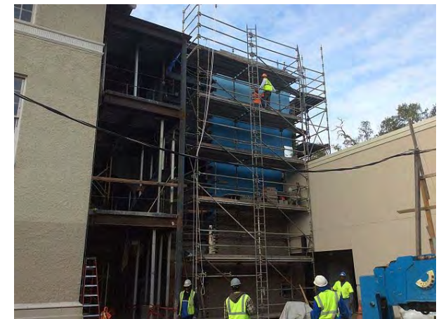
Audubon School Renovation Construction 85% Complete
