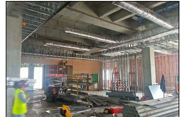
Alfred Lawless School Interior & Mechanicals Construction Ongoing
