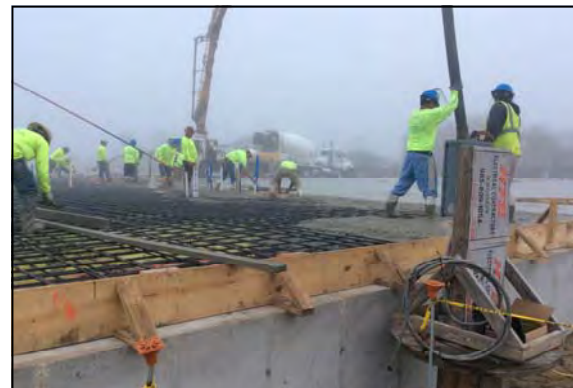
Carver High School—Design/Build Foundations Poured
