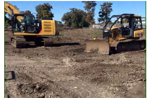
Paul B. Habans School Design/Build Site Preparation Underway
