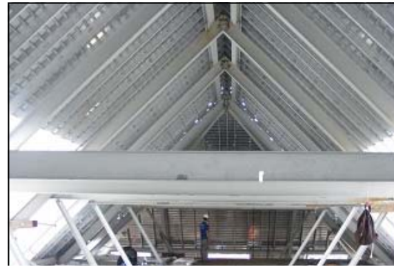
Andrew J. Bell—Roof Replacement Construction Nearly Complete
