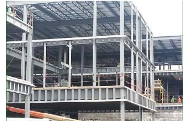
Fisk-Howard School Steel Erection Ongoing
