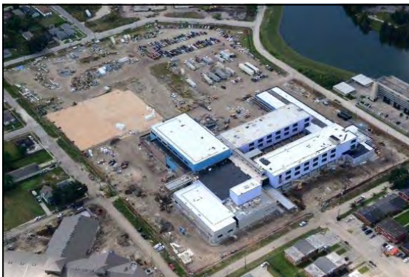
McDonogh 35 (Phillips/Waters) High School Construction Continuing On Schedule
