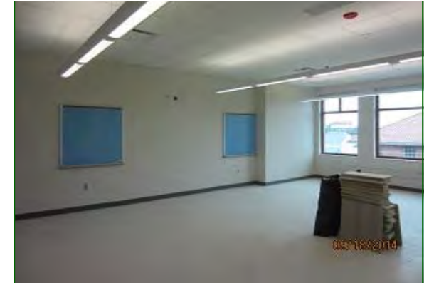
Fisk-Howard Pk-8 School Construction Nearly Complete
