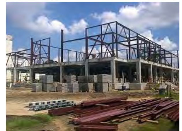
Eleanor L. McMain Gymnasium Structural Steel Erection In Progress
