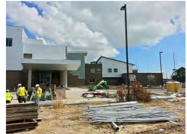
Edward Livingston High School Finishes and Flooring Installation Ongoing
