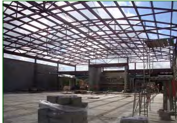
Lake Forest School at Greater St. Stephens Structural Steel Erection Progressing
