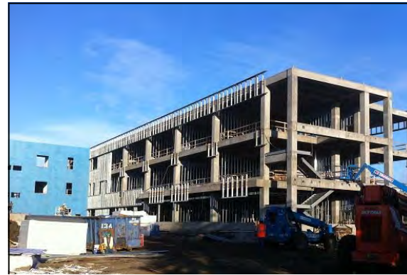
Stuart R. Bradley School Steel and Wall Construction In Progress
