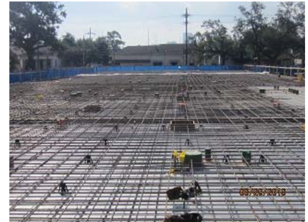
Fisk-Howard School Foundation & Steel Erection Begun
