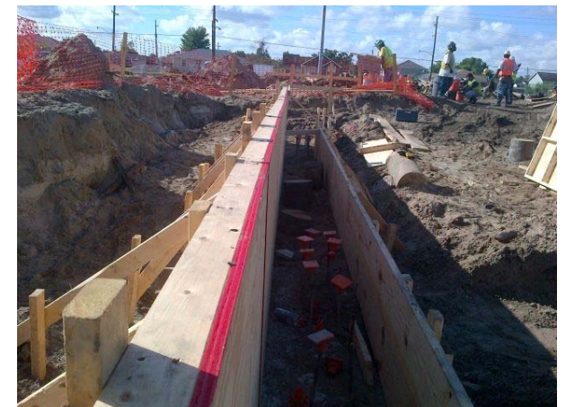
Edward Livingston High School Foundation Work In Progress
