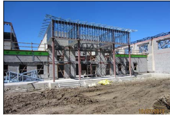
Alice Harte PK-8 School Masonry & Steel Erection in Progress
