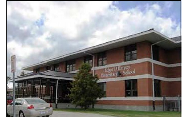
Edgar P. Harney Elementary School Refurbishment Design Started
