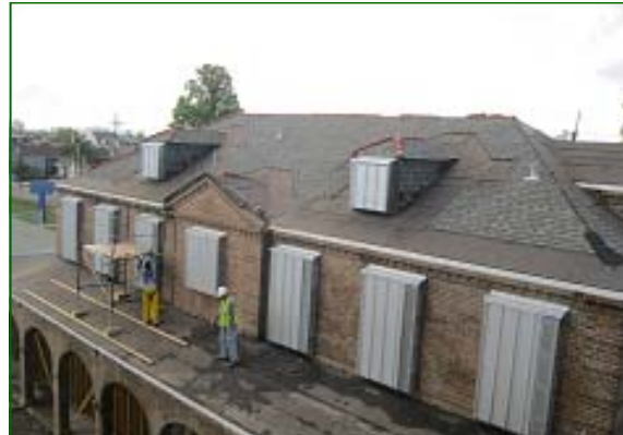
Andrew J. Bell—Safe & Secure Moisture Control & Roofing Underway
