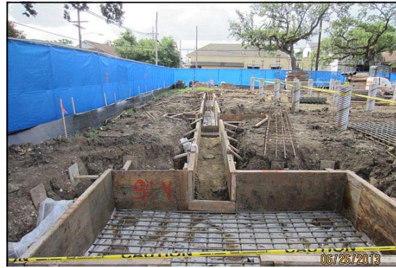
Fisk-Howard New Construction Piles and Foundation Work Progressing
