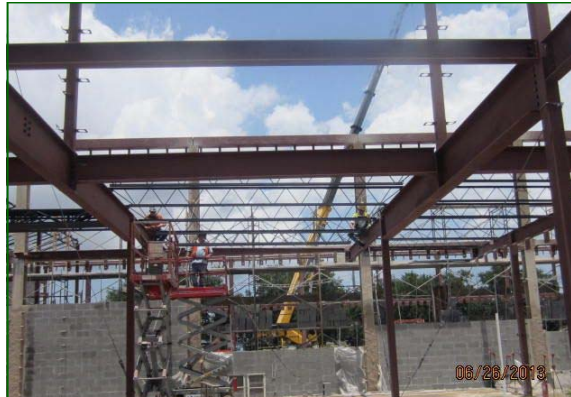
Alice Harte Elementary Steel Erection in Progress
