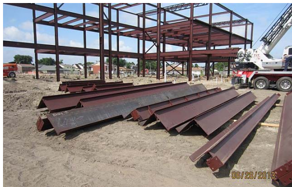
New PK-8 School at North Kenilworth Park Steel Erection Begun
