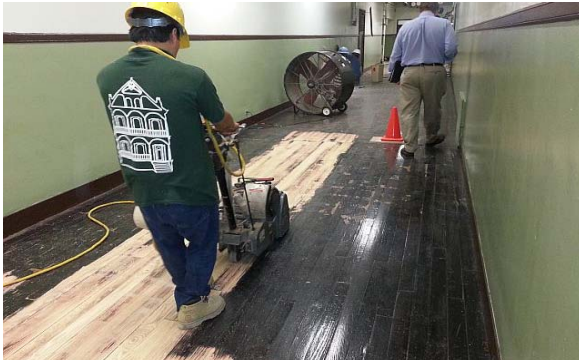
Frederick A. Douglass H.S. Refurbishment Floor Repair & Refinishing In Progress
