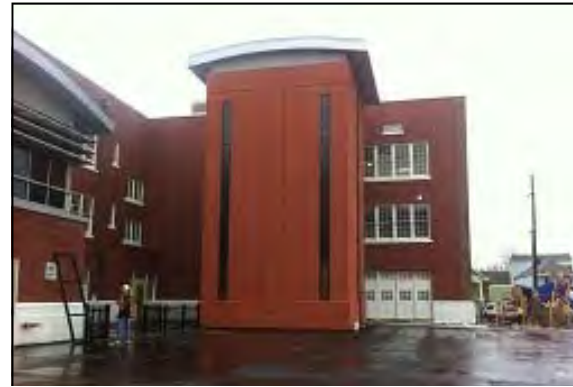
Drew Elementary School Renovation Substantial Completion in April 2015
