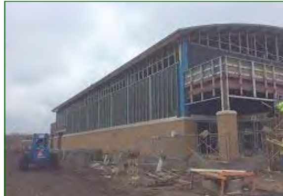
Lake Forest School at Greater St. Stephens Substantial Completion In May, 2015
