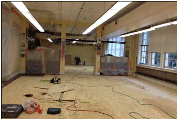
Warren Easton High School Interior Refurbishment Progressing
