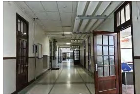
Frederick A. Douglass High School New Windows & Painting In Progress
