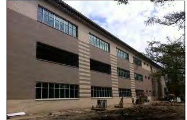
Alice Harte School- Construction Complete in Fall 2014
