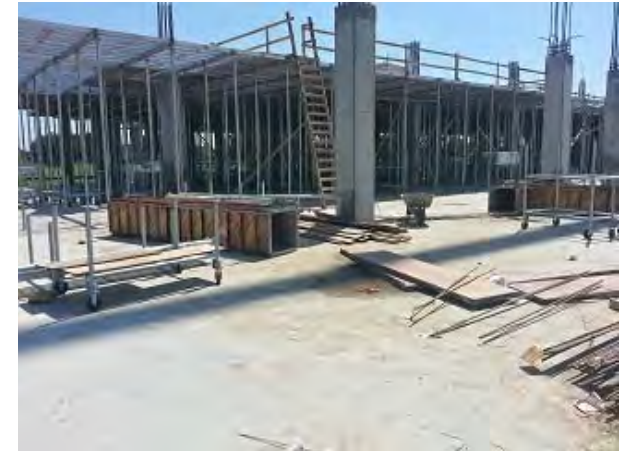
Alfred Lawless High School Steel Erection Underway
