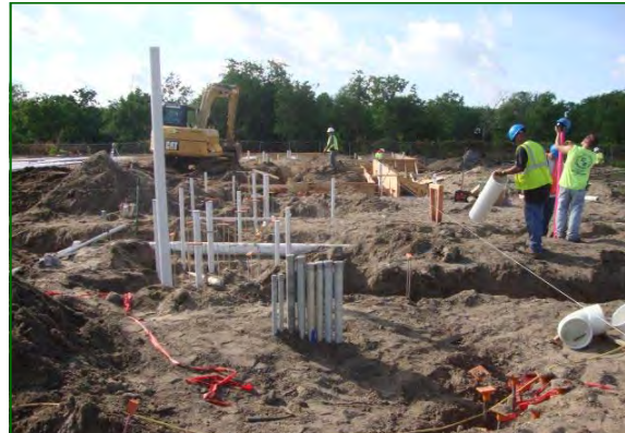
Lake Forest School at Greater St. Stephens Construction Progressing
