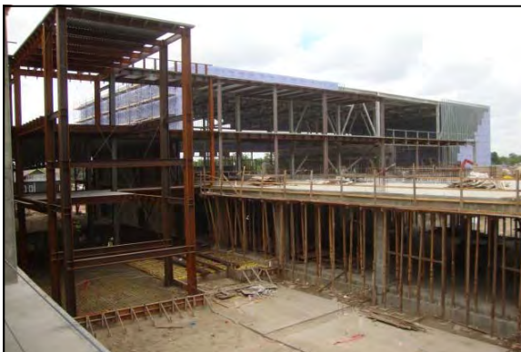
McDonogh 35 (Phillips/Waters) High School Construction 50% Complete
