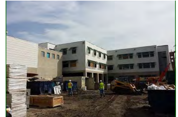
Fisk-Howard Pk-8 School Interior Mechanicals Being Installed
