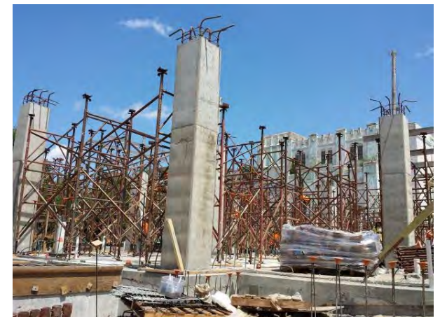
Eleanor L. McMain Gymnasium Structural Piles and Floors Being Poured
