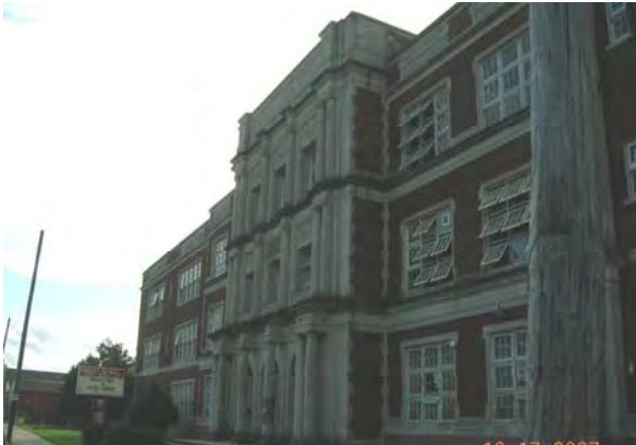
Existing Colton Building
