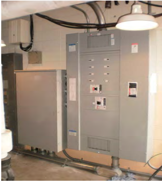
Banneker Elementary after repairs
