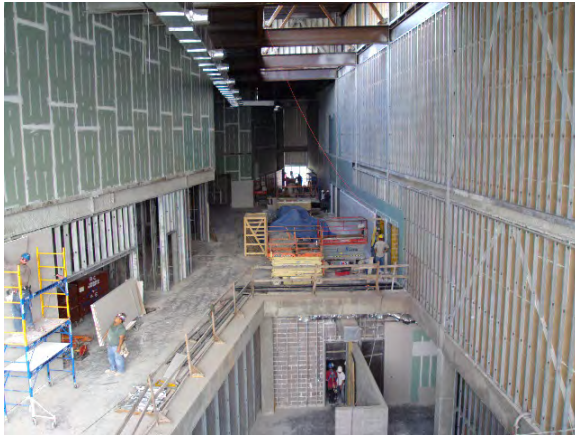
L B Landry-Ongoing Construction
