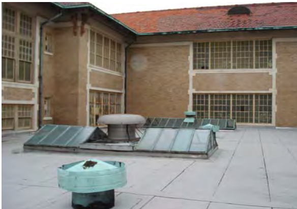
Existing roof at Live Oak ES
