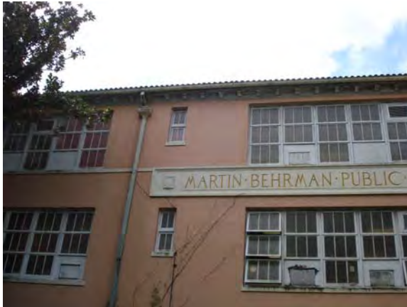
Behrman ES before replacement of roof
