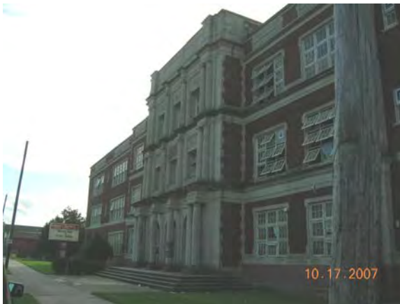
Existing Colton facility
