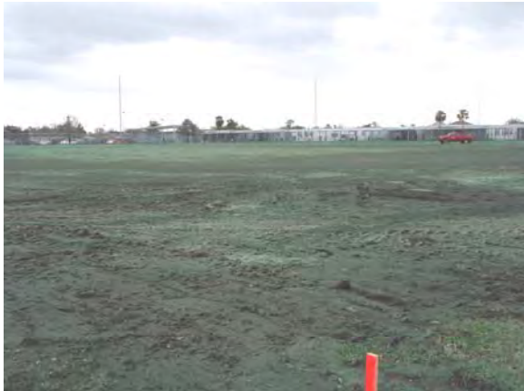
Fannie C. Williams Demolition Complete
