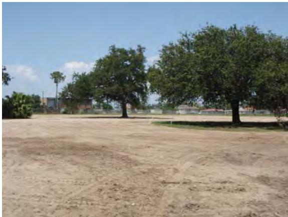
Parkview Demolition complete
