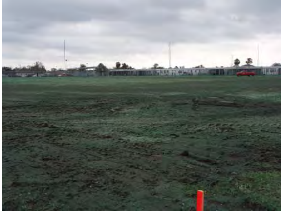
Fannie C. Williams Demolition Complete
