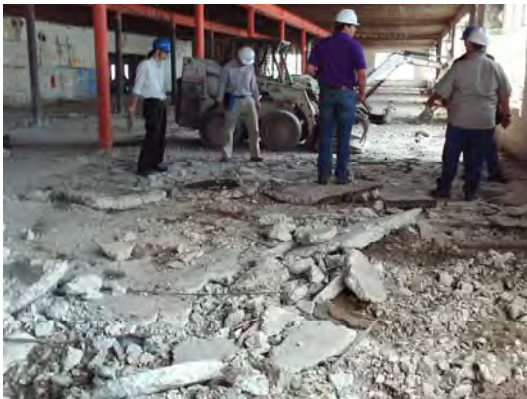
Interior demolition continues at Craig Elementary
