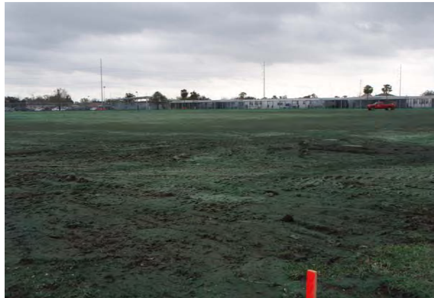
Final photo of Fannie C Williams site after demolition was completed.
