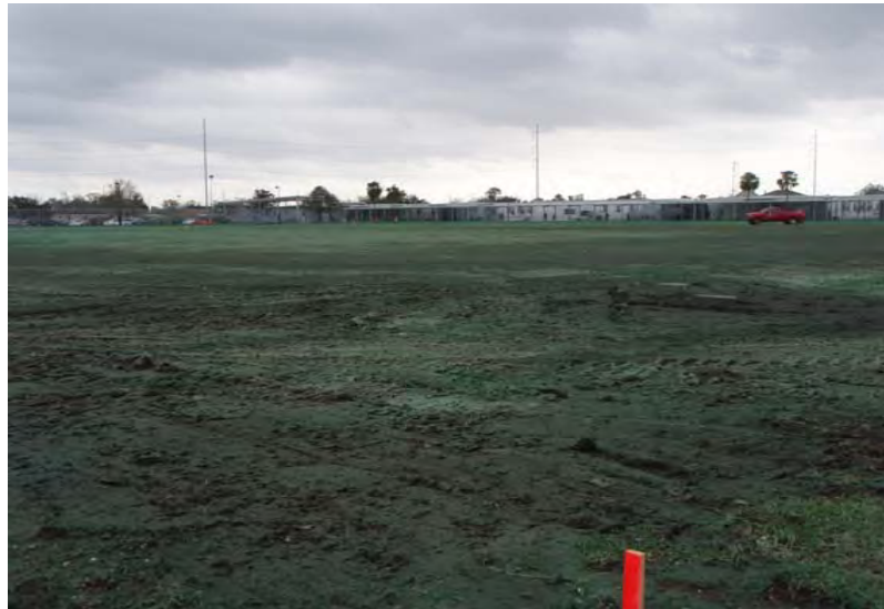
Final photo of site after demolition was completed.
