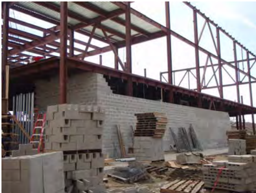
Structural steel on the 2 nd half of the new building at Andrew Wilson Elementary
