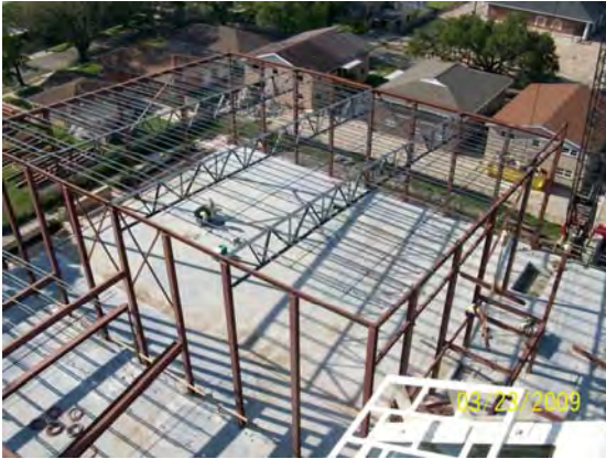
Structural Steel at Lake Area
