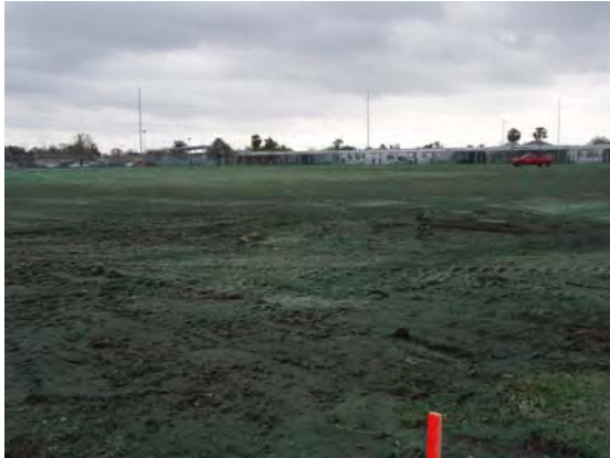
Final photo of Fannie C Williams site after demolition was complete
