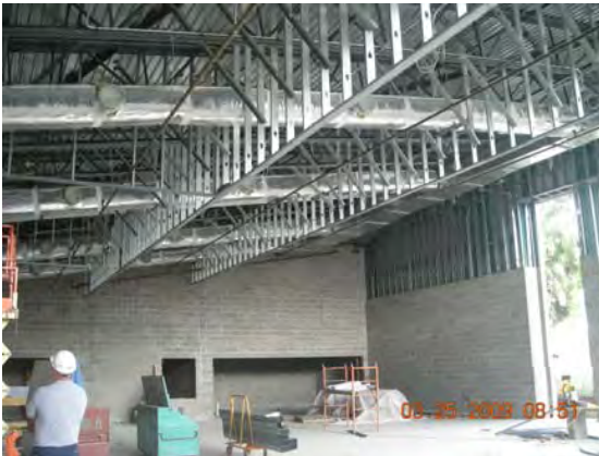
Masonry block wall assembly continues at Langston Hughes
