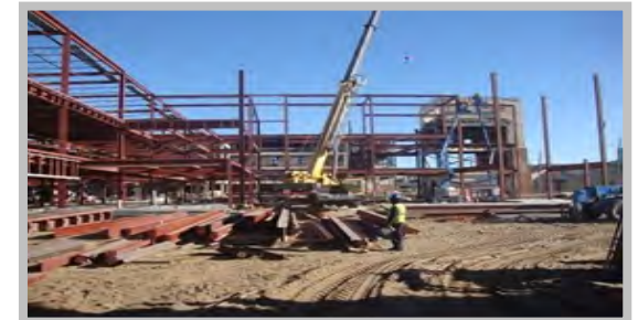
Booker T. Washington High School Construction Continuing
