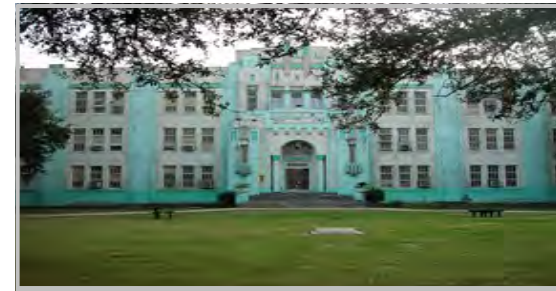
Eleanor McMain School Envelope Repairs
