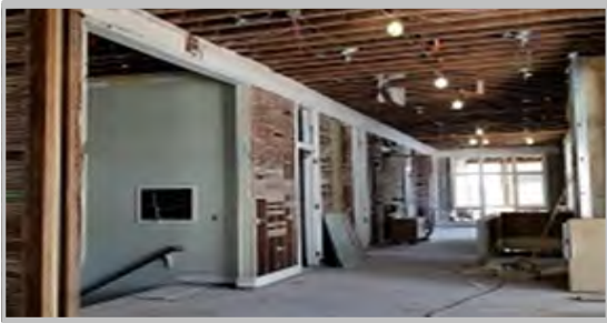
Harriet R. Tubman Elementary School Renovation Continuing Construction
