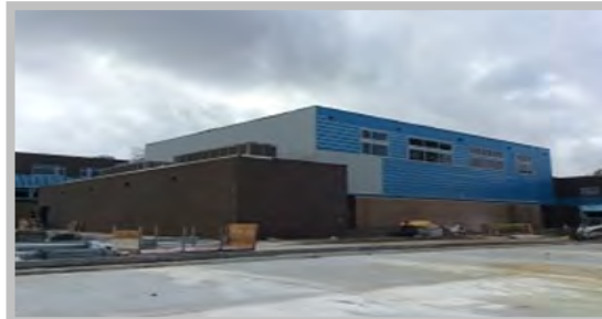
Paul B Habans School Construction Continuing
