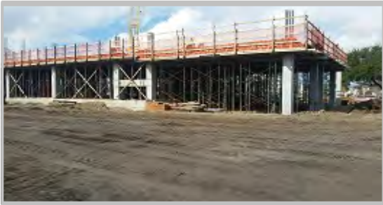
Avery Alexander Elementary School Construction Continuing
