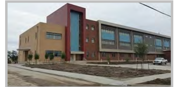
Alfred Lawless School Substantial Complete December 2015
