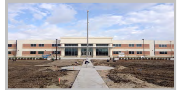
George Washington Carver High School Construction Continuing
