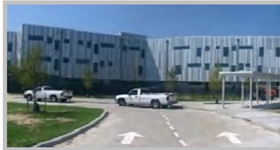
New PK-8 at North Kenilworth Park Construction Continuing
