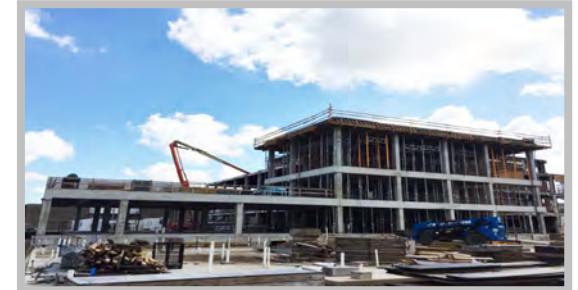
Booker T. Washington High School Construction Continuing
