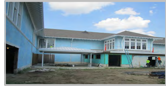
Harriet Tubman Elementary School Renovation
