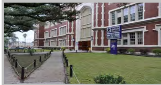
Warren Easton Waterproofing Construction Continuing
