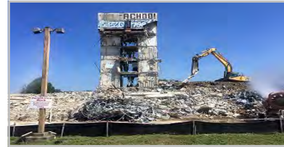
JoEllen Smith Medical Center Demolition
