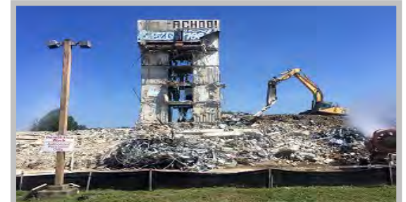
JoEllen Smith Medical Center Demolition Demolition Nearing Completion
