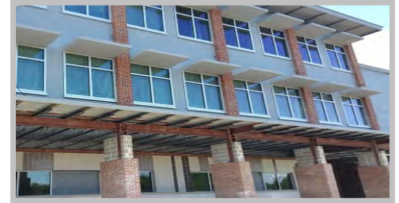
Ernest "Dutch" Morial Elementary School Construction Continuing
