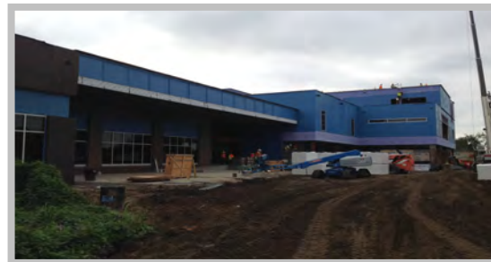
Paul B Habans School Construction Continuing
