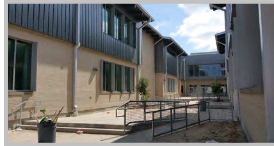
Small New Orleans East High School at Abramson Substantial Complete September 2015
