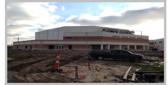
George Washington Carver High School Construction Continuing
