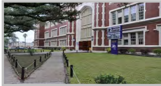
Warren Easton Waterproofing Construction Continuing
