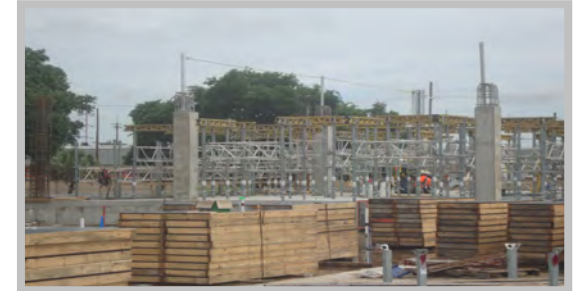
Booker T. Washington High School Construction Continuing
