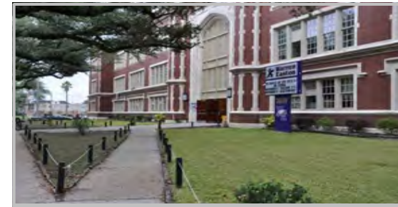
Warren Easton School Courtyard Waterproofing
