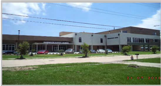
Paul B. Habans School Substantial Complete June 2016
