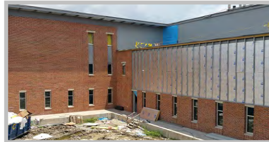
Paul B Habans School Construction Continuing
