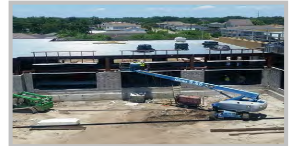
Avery Alexander Elementary School Construction Continuing
