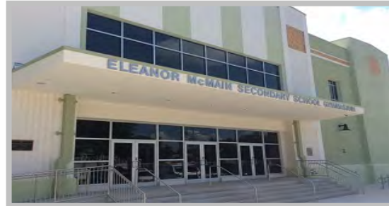
Eleanor L. McMain School Gymnasium Substantial Complete June 2016
