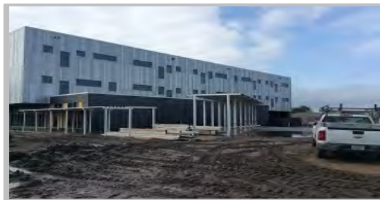
New PK-8 at North Kenilworth Park Construction Continuing
