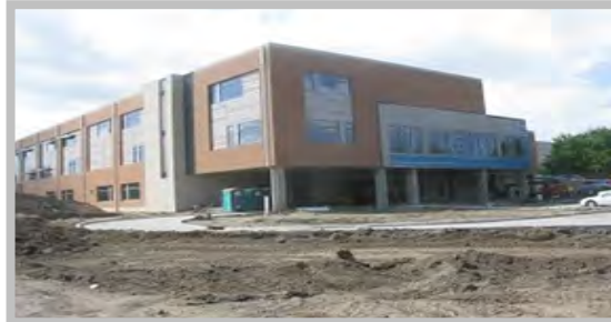
Avery Alexander Elementary School Construction Continuing
