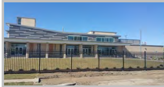
Ray Abrams Elementary School Substantially Complete
