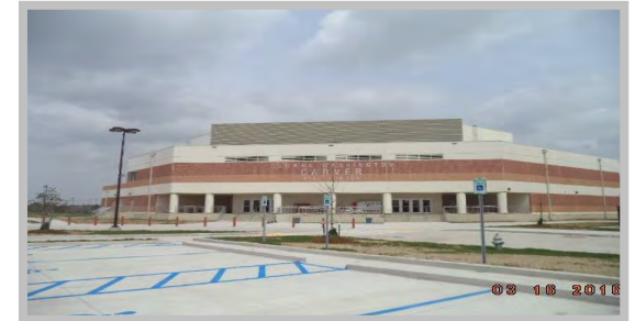
George Washington Carver High School Substantial Complete March 2016
