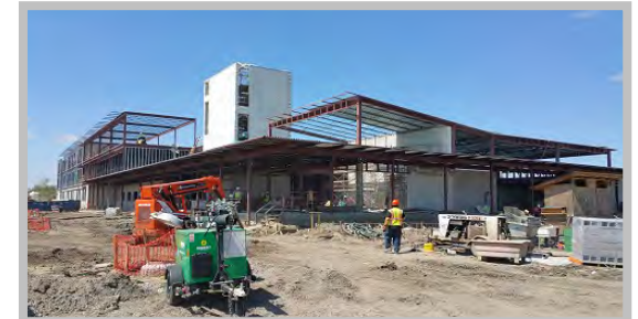
Ernest "Dutch" Morial Elementary School Construction Continuing
