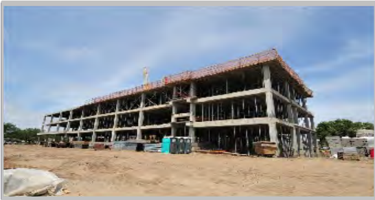
Avery Alexander Elementary School Construction Continuing
